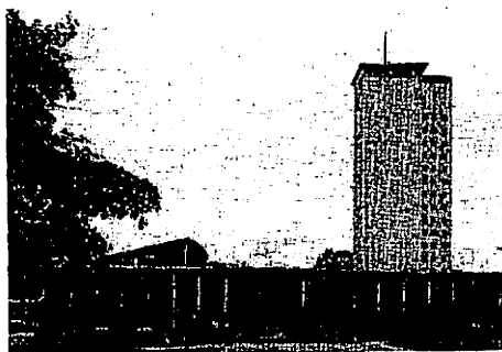
Fig. 1 Administration Block, Univ. of Ibadan, by M. Fry, J. Drew et al. (1953-59), Ibadan, Nigeria (Photo: author)
