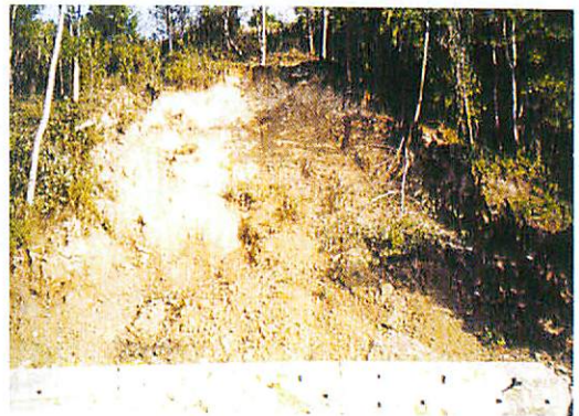
Fig. 6 Bioengineering site B4 at chainage 1+530 km view towards east
