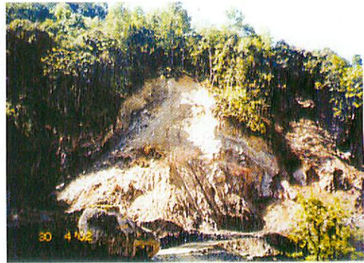
Fig. 9 Bioengineering site B1 at 6+400 km view towards east
