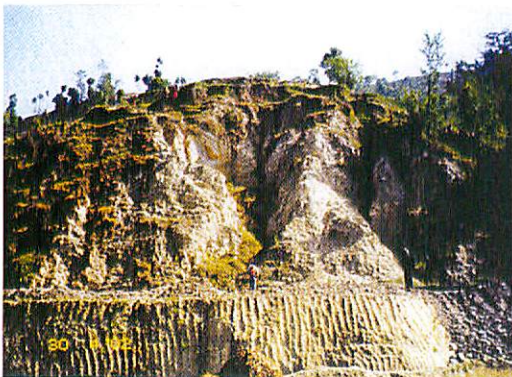
Fig. 5 Bioengineering site B3 at chainage 1+000 km, view towards north
