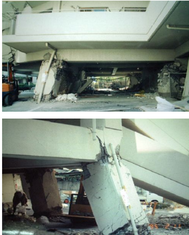
Fig1.2 Pilotis RC building damaged by flexural failure in Hyogoken-nanbu EQ (M=6.7), Hiroshima, 2001
