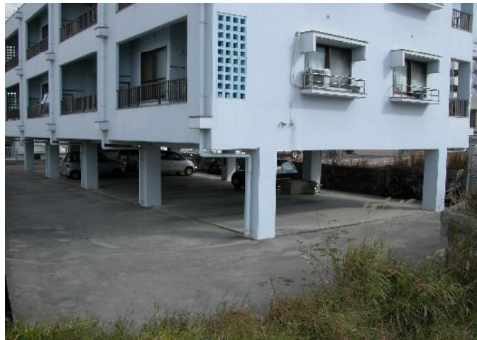
Fig. 4.6 An existing soft-first-story building
