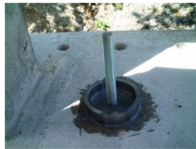
Fig. 2.7 Detail of disk-anchor (unit:mm)
