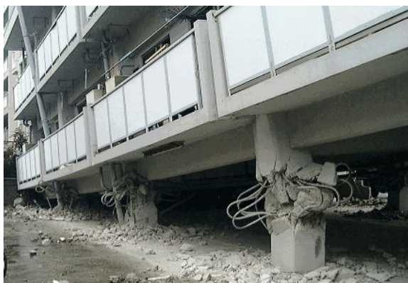
Fig. 1.1 Pilotis RC building damaged by shear-compression failure in Geiyo EQ (M=6.7), Hiroshima, 2001
