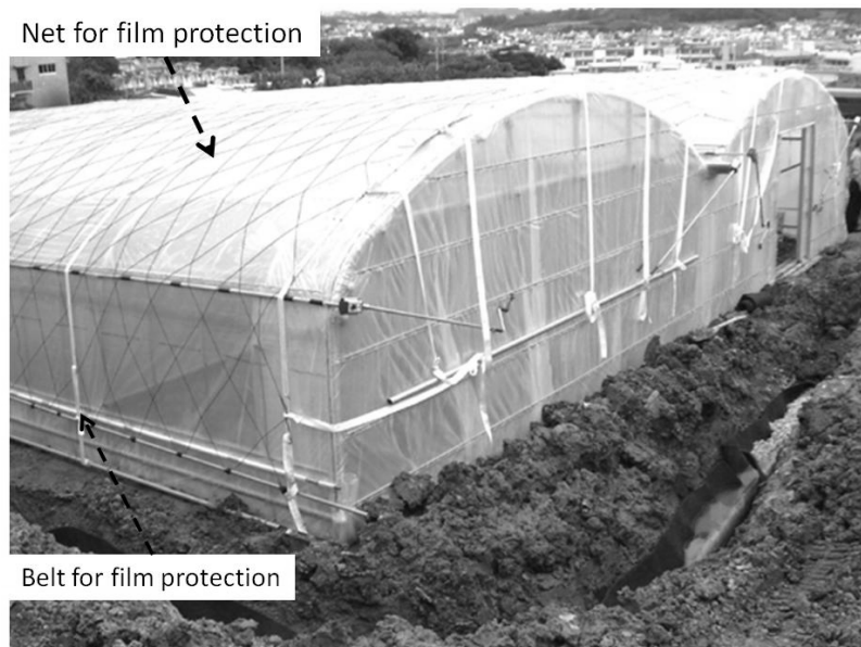
Fig. 4.3. Installation of net for film protection.
