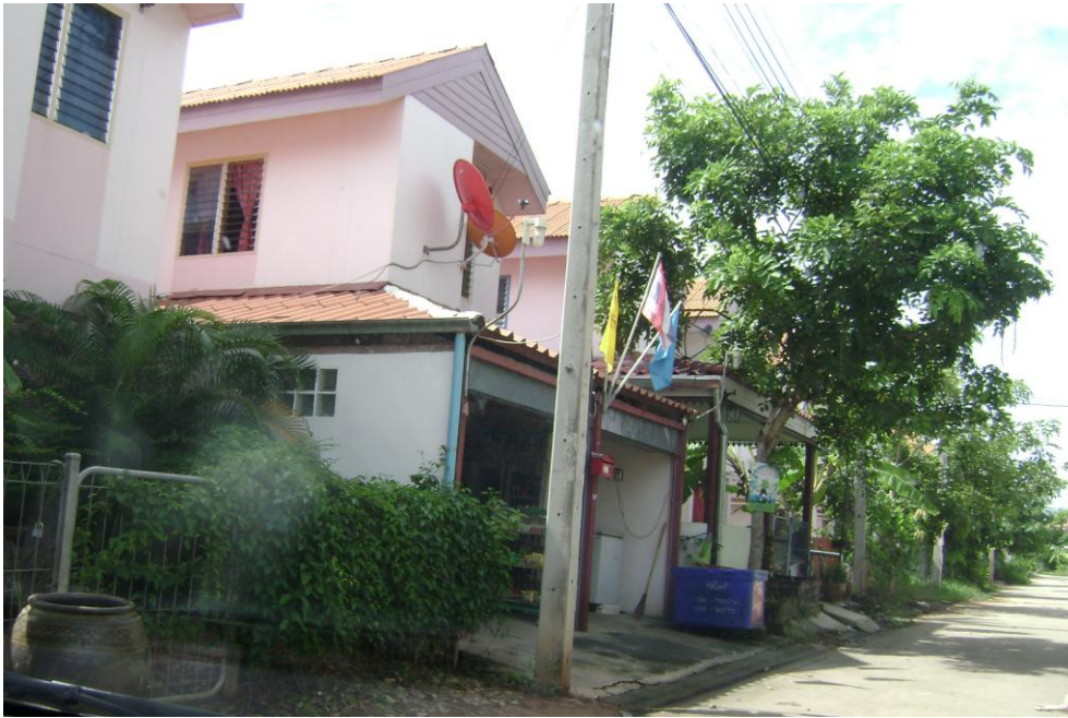
Fig. 2.2 Nationwide Low-cost Housing Project Characteristics with Its Extended Low-income Generation Space Capability
