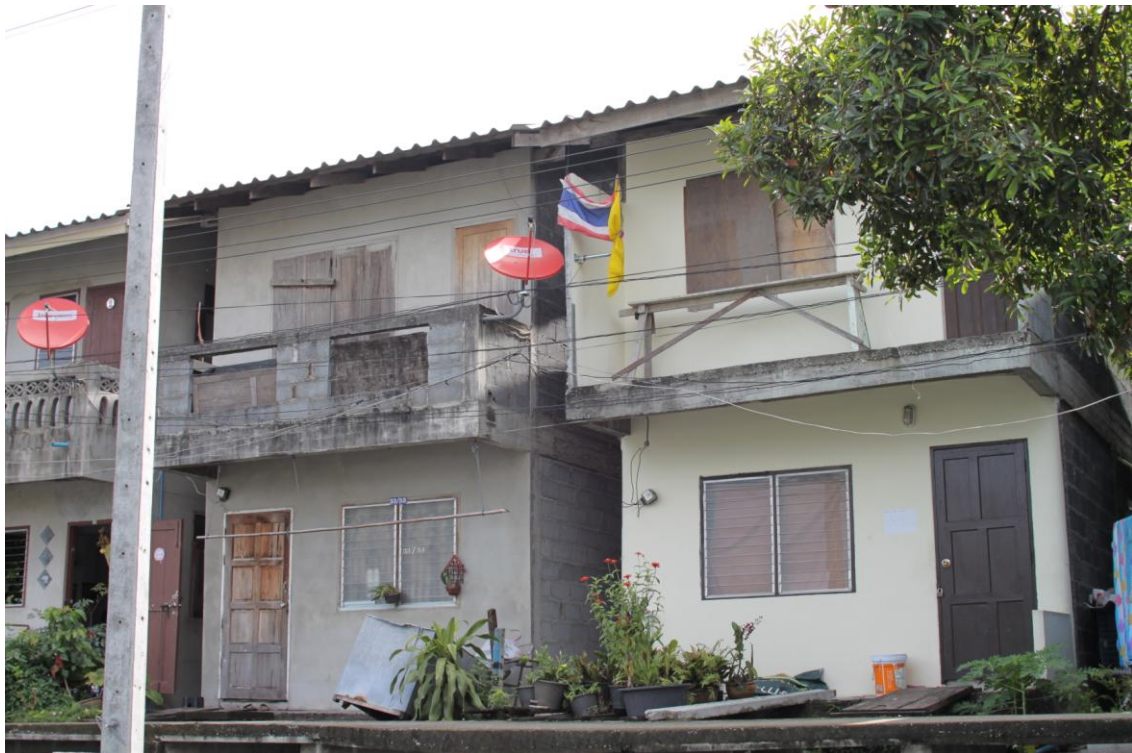
Fig. 3.3 Photograph of Unpainted House and Under Painting Process House
