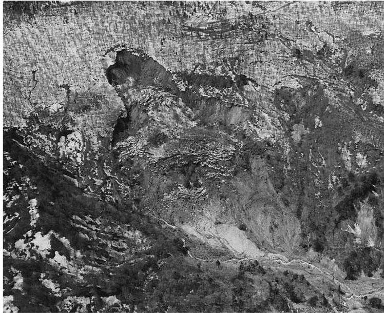
(a) The aerial view of landslide in Akita (from 小野ら 2006)
