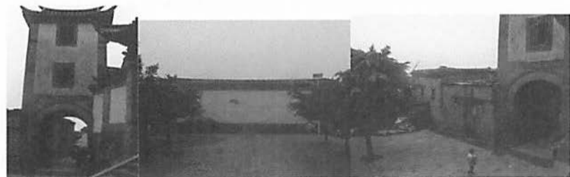
Tower gate and screen wall
