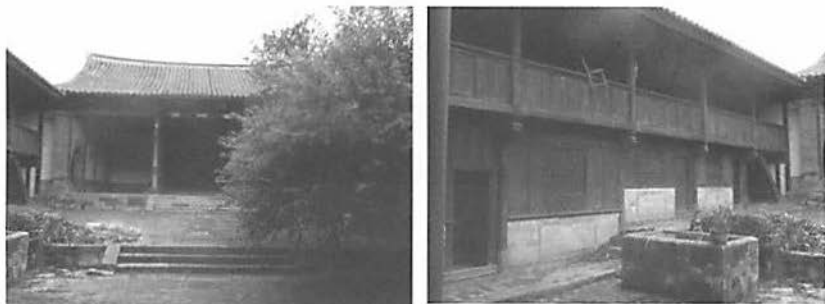
Main room and side room
