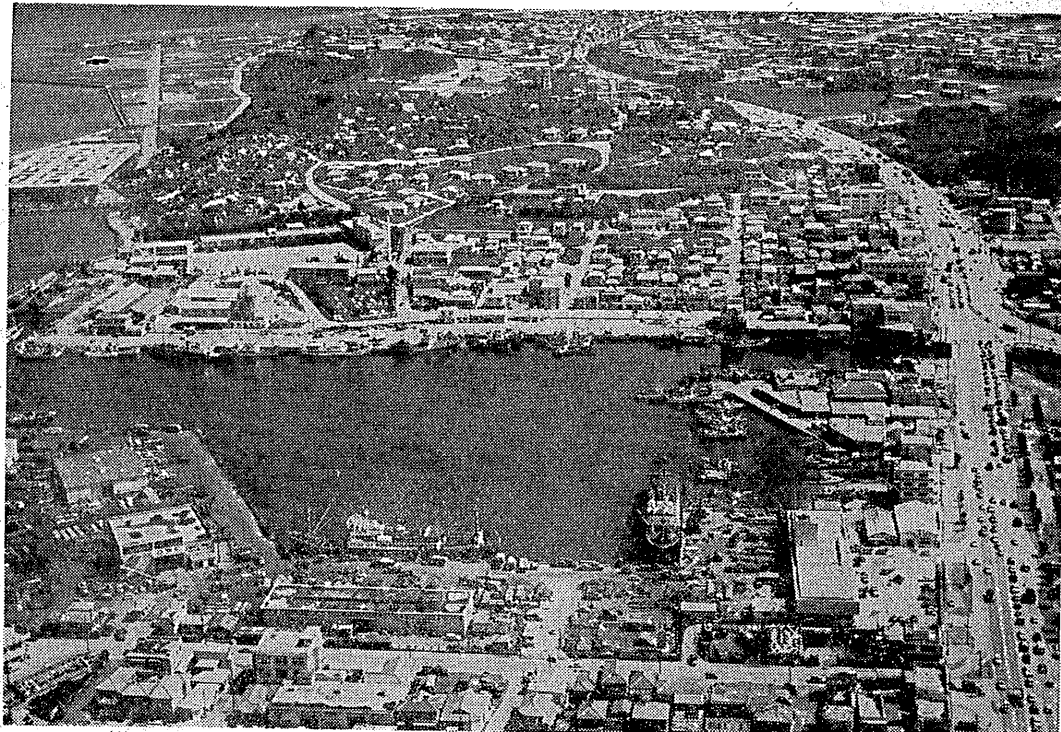
OKINAWA PORT—Tomari Port, expanded in 1953 from a tiny fishing cove, handles bulk of shipping between the Ryukyus and mainland Japan by small freighters, passenger ships and others up to 2000 tons each.
