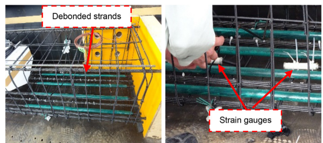
Fig. 21. Debonded strands and strain gauges at end of girder.
