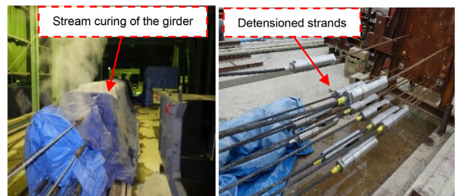
Fig. 22. Steam curing and detensioning process.
