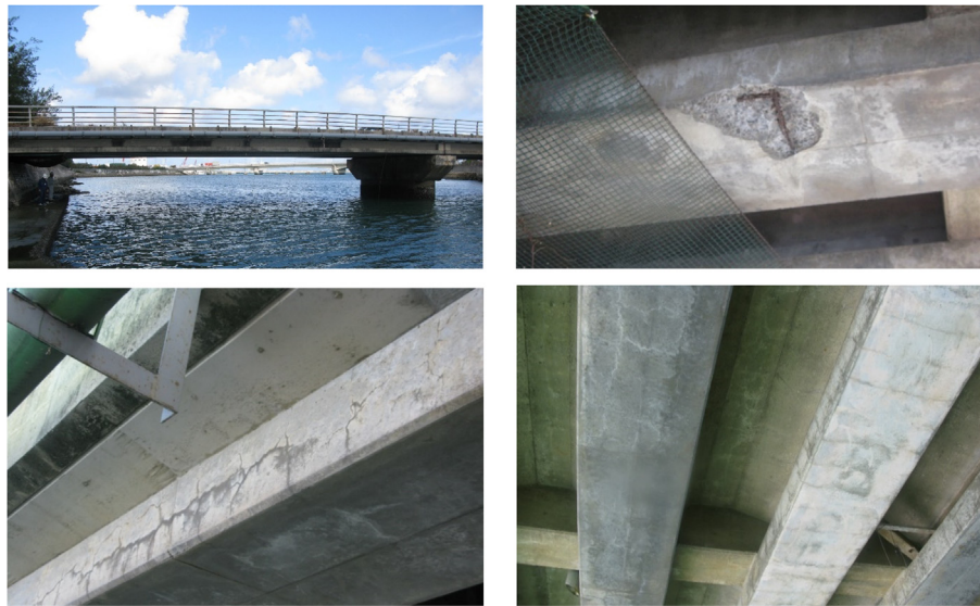
Fig. 1. Deteriorated preflex beam bridge.
