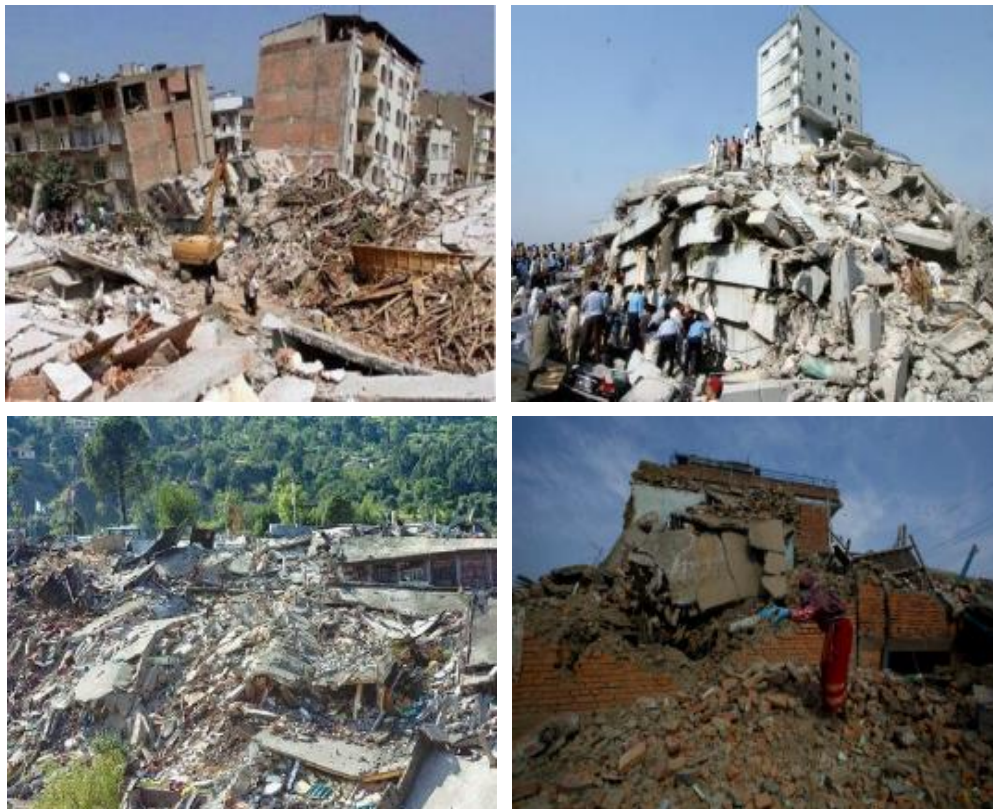
Figure 6.12 Destruction of reinforced and masonry structures in 2005 Mw 7.6 Kashmir earthquake
