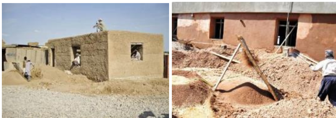
Figure 6.6 Houses made of stack wall: Left: Room ready for roof construction. Majority of the houses in Nahrin of Baghlan province has the same structure with some recent addition of wooden pools within the walls. Right: Mud preparation for plastering of stack walls.
