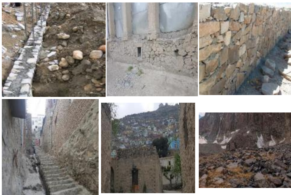
Figure 6.4 Stone masonry, Left to right: Continuous footing between concrete columns, foundation of an old structure in the outskirts of a hill in a central area of Kabul city, near Shah-e-du shamshira Masjid, dry stone masonry work which are still taking place on large scale, a stone masonry work for foundation of a residential building in a hillside in central Kabul, a view of relatively new built houses in hillside in Kabul and abandoned rocks available in a mountain.
