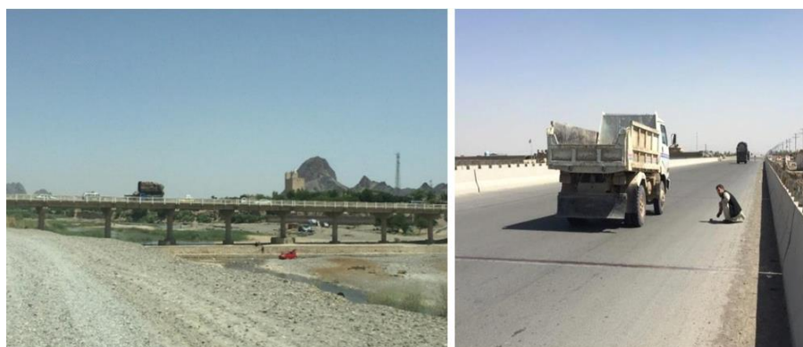
(a) Bag-e-Pul Bridge
