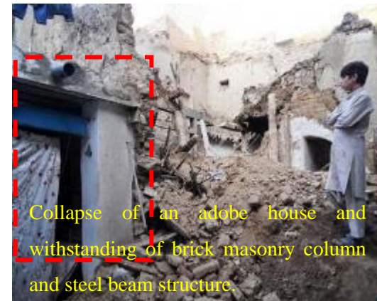
Figure 6.11 Illustration of collapse mechanism of the adobe, mud-brick and stone masonry structures in Nahrin and Rustaq earthquakes of Afghanistan.
