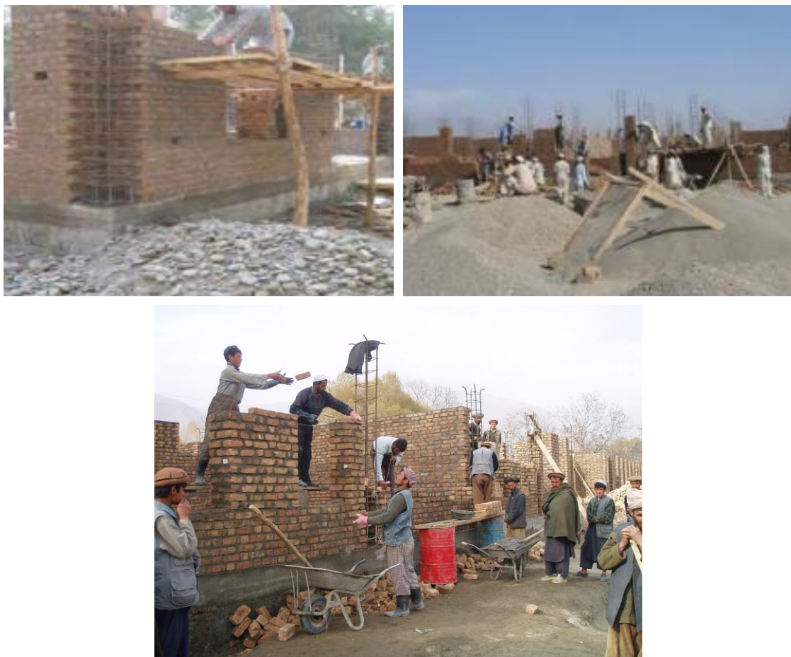
Figure 6.9 Example of construction of brick masonry walls in Afghanistan.
