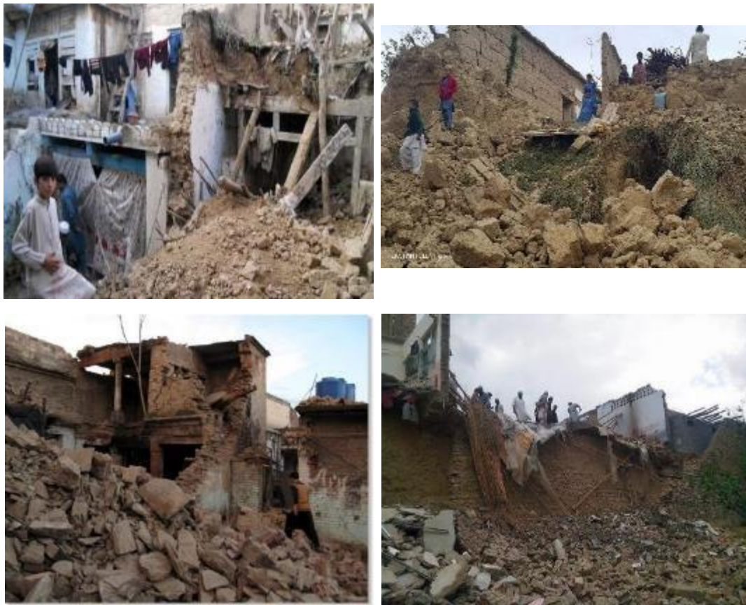
Figure 6.14 Collapse mechanisms of adobe structures in 2015 Hindu Kush earthquake of Afghanistan and Pakistan.
