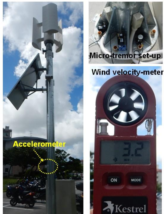
Figure 8.34 View of the pole and instrumentation
