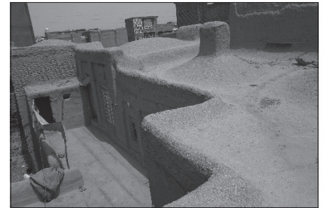
Fig. 2 Traditional house with domical vault roofs in Herat (Photograph by K. Kawish 2016)
