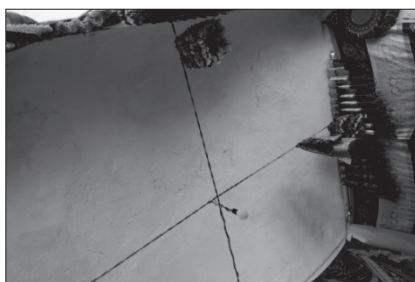
Fig.17 Tie-bars on ceiling of living room- Ahmad house (Photograph K. Kawish 2016)
