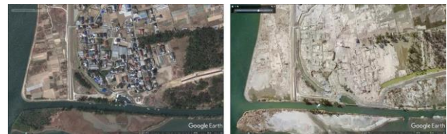
Photo 4 Damages of the residential area where there was little coastal forest on the seaside front of it. (location ①)
