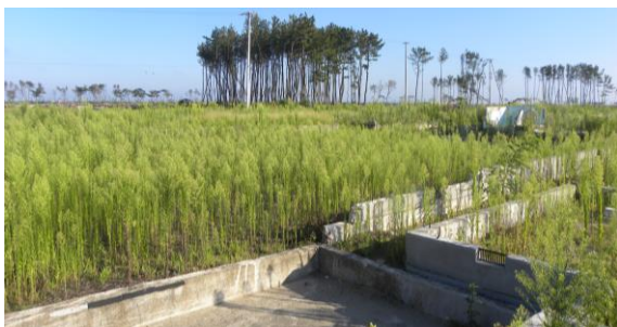
Photo 2 The state of the most of the houses swept away, and left only its foundation parts. In the distance, several trees of the forest that endured against the tsunami can be seen.
