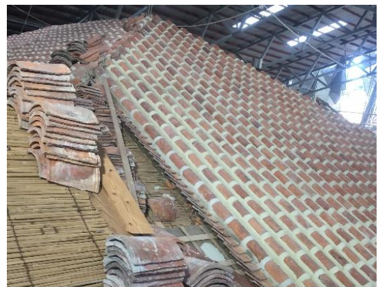
Photo 2 Red tile roof under repairing
