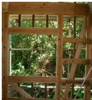
Photo 3 Framework (Nuki only) Photo 4 Framework (Nuki+brace)
