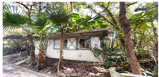
Fig. 12. Pump operation room existing before the campus relocation.
